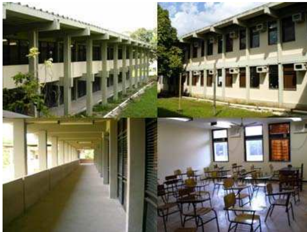
Fig. 1. Photograph of the building. In clockwise: external side with glass windows, classroom, corridor and external side with corridor along
